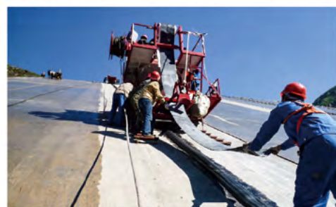
Mechanized installation of GB waterstop materials
